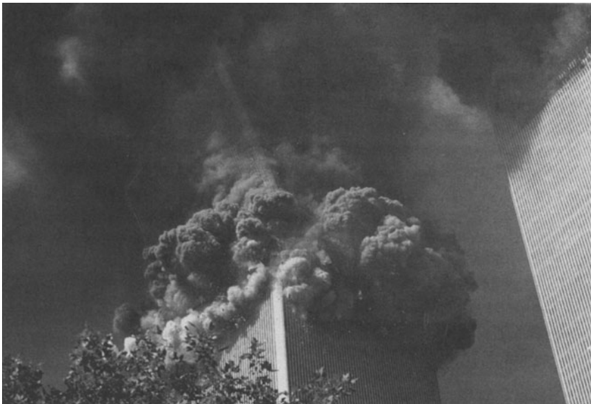
Figure 1.2. The collapse of World Trade Center Tower 2. Courtesy of Thomas Nilsson/Getty Images
